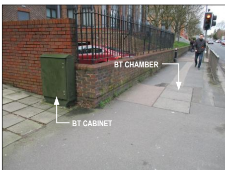
PHOTOGRAPH 1 EXISTING BT CABINET AND CHAMBER ON WEST SIDE OF LONDON ROAD TO SOUTH OF BUILDING
