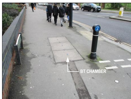
PHOTOGRAPH 2 EXISTING BT CHAMBER IN FOOTWAY ON WEST SIDE OF LONDON ROAD TO SOUTH OF BUILDING
