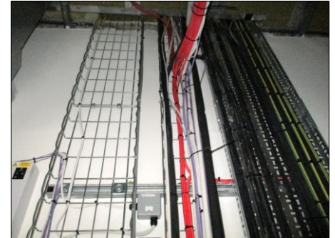
PHOTOGRAPH 15 TYPICAL VIEW OF TELECOMS RISER ON GROUND FLOOR INDICATING AVAILABLE SPACE TO UPPER FLOORS
