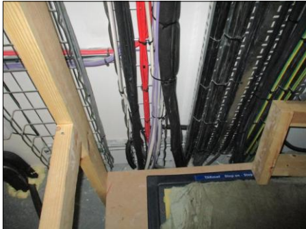
PHOTOGRAPH 13 TYPICAL VIEW OF CABLE ENTRY INTO RISER ON GROUND FLOOR FROM BASEMENT PARKING AREA
