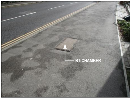
PHOTOGRAPH 4 EXISTING BT CHAMBER IN FOOTWAY ON LONDON ROAD OUTSIDE BUILDING
