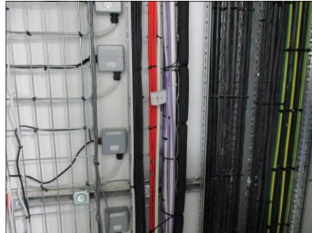
PHOTOGRAPH 14 TYPICAL VIEW OF EXISTING TELECOMS SERVICES IN RISER ON GROUND FLOOR TOWARDS CENTRE OF BUILDING
